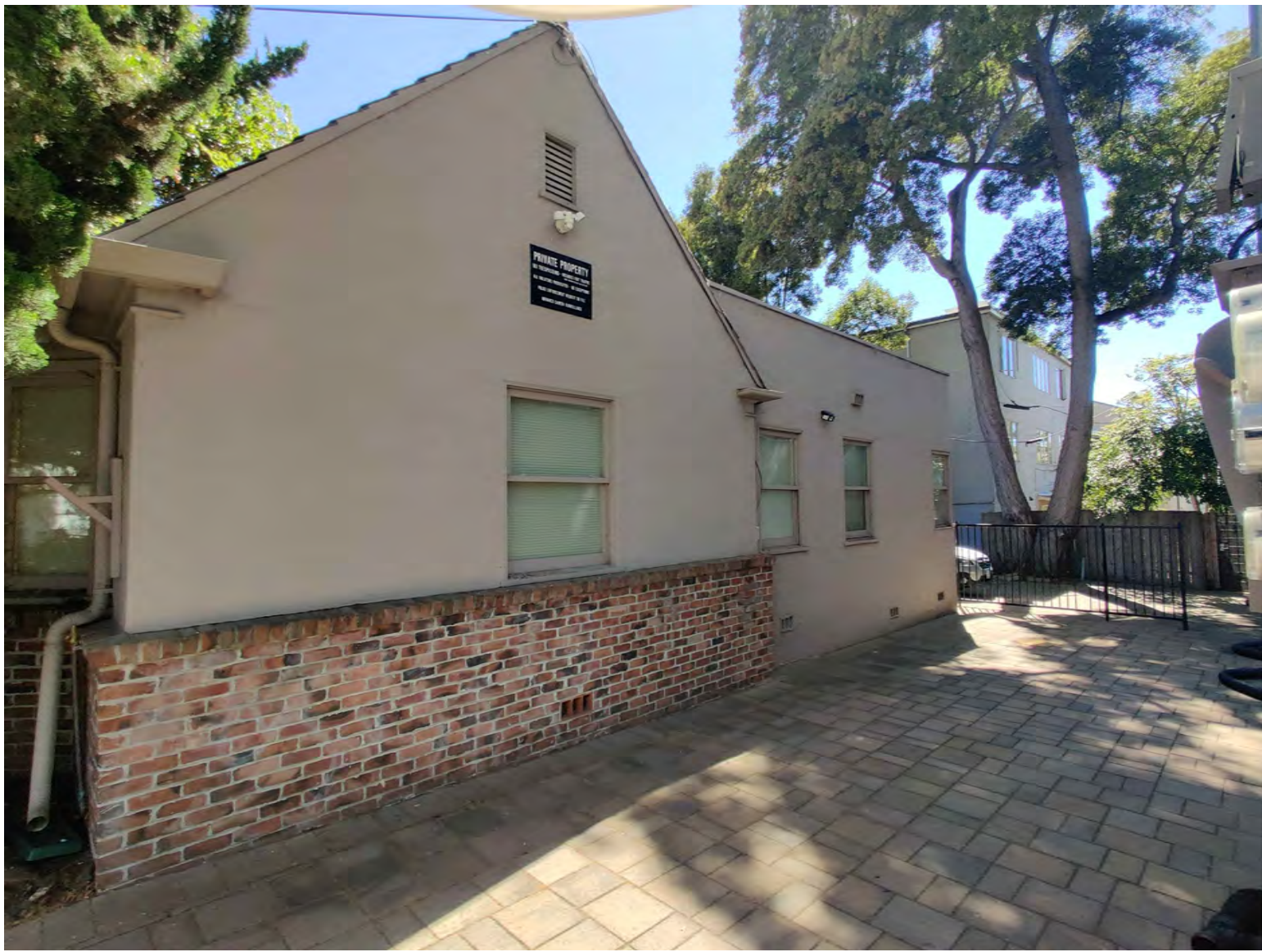
6 LOOKING S AT N FACADE OF 2241 CHANNING
