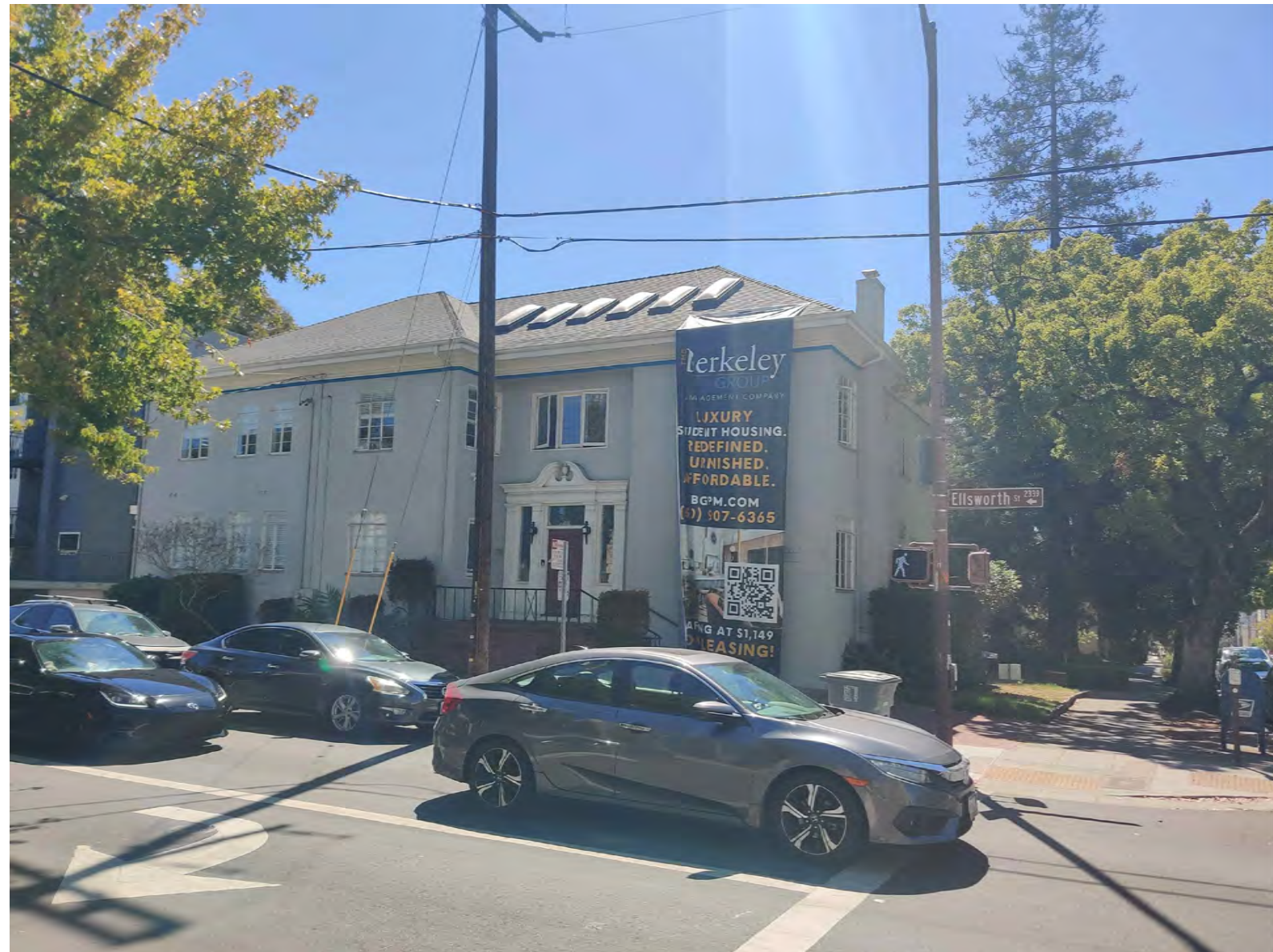
1 LOOKING SW FROM STREET CORNER
