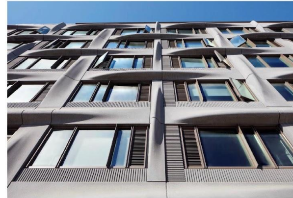
TOWER FACADE: GFRC
