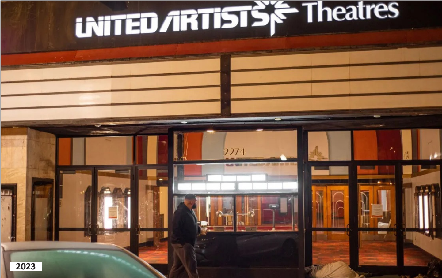
Entry before temporary panels installed.
