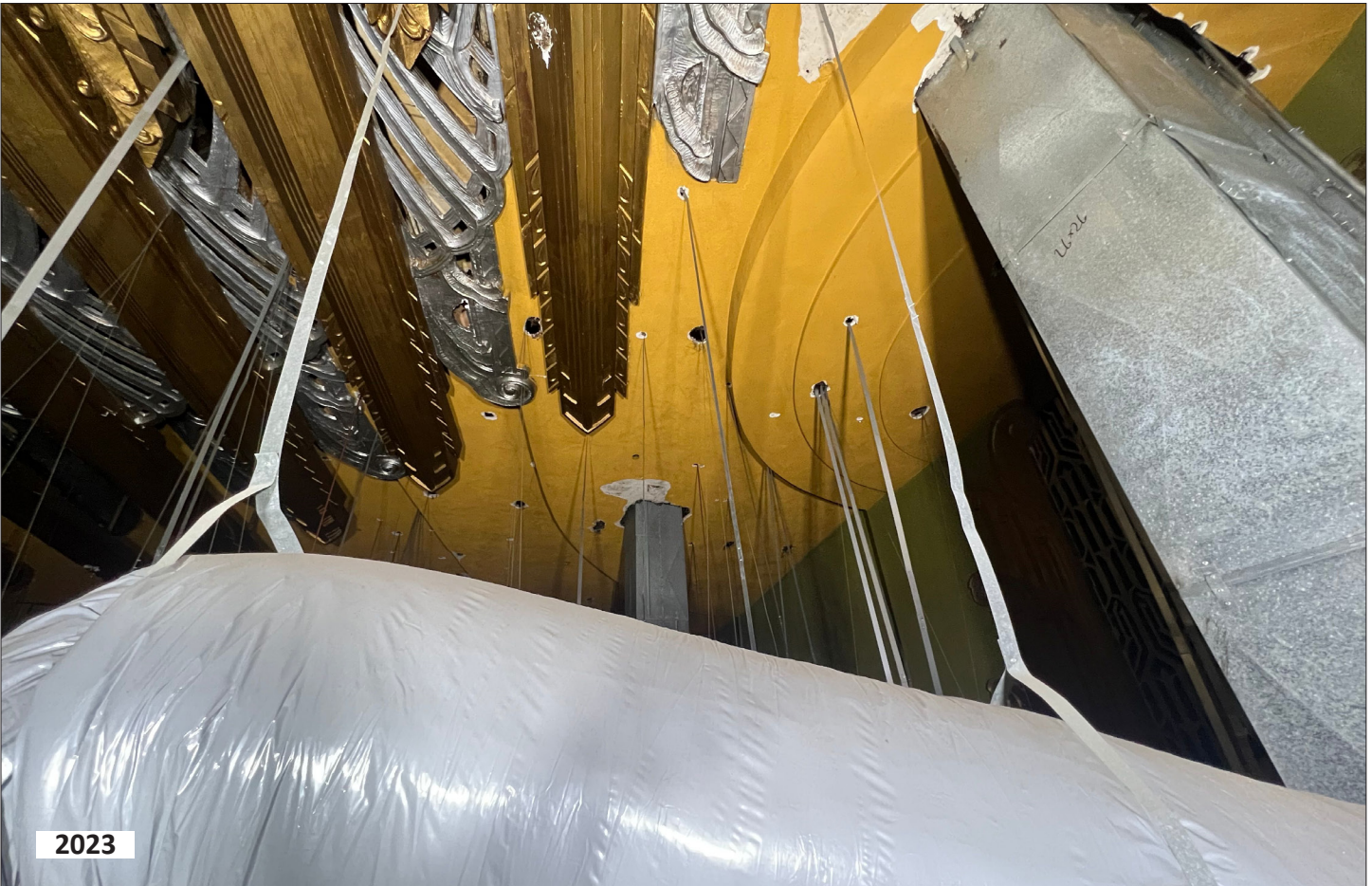
Ceiling & stage proscenium (after alteration): remaining remnants with suspended ceiling & HVAC
