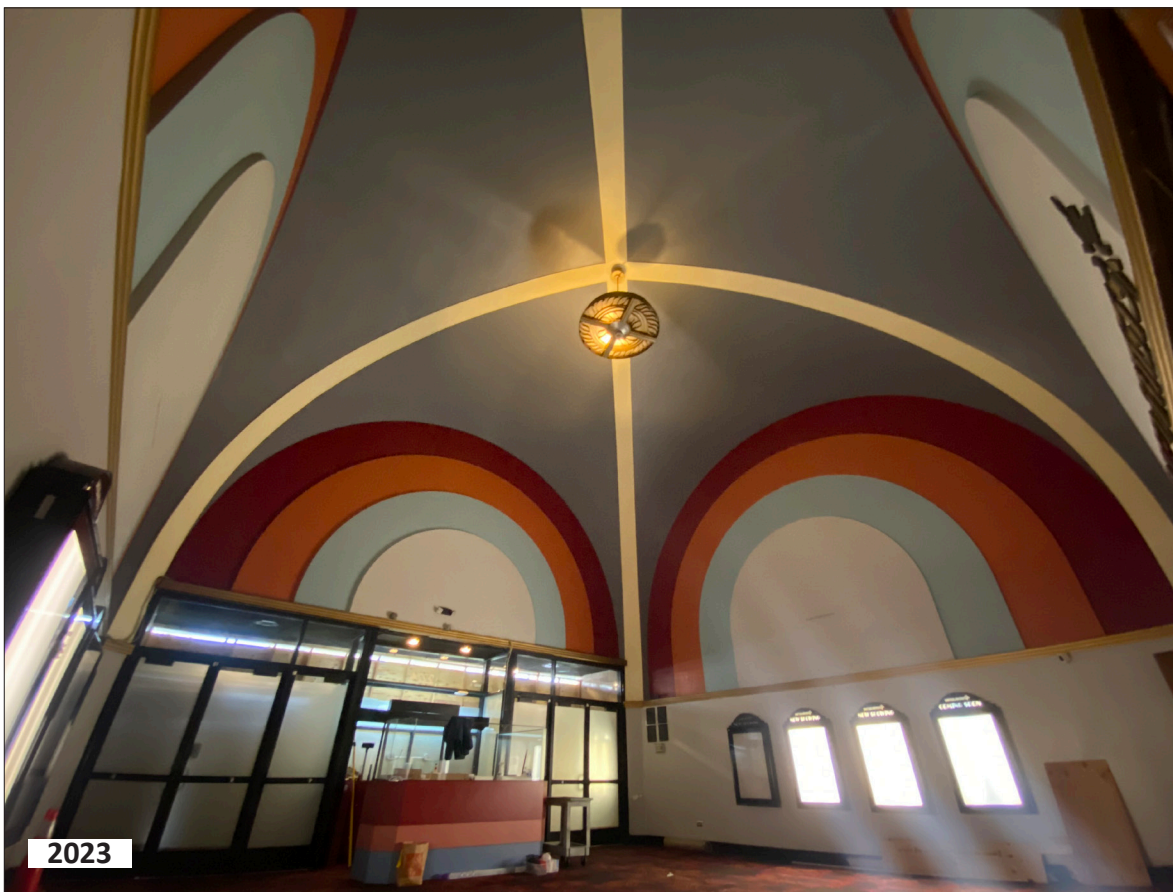
Atrium, looking southeast. The tiled walls & pavement have been removed.
