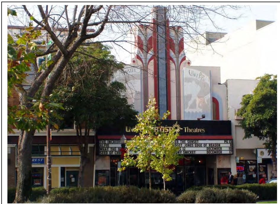
Photograph 1. United Artist building, camera facing west, November 16, 2004.
