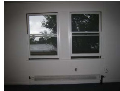
IMG_7109 baseboard radiator below paired double hung windows as in original dormitory rooms
