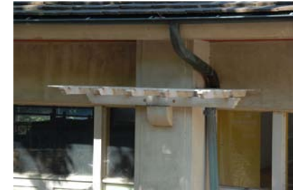
DSC_0024 wood trellis and copper gutter and downspout, east elevation
