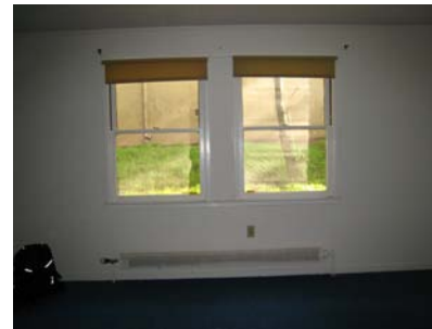
IMG_7039 paired double hung windows with radiator below
