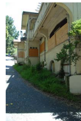
DSC_0090 curved plaster brackets below balcony
