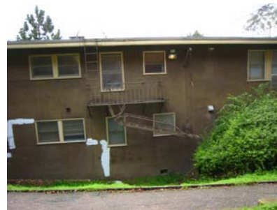
IMG_7067 fire escape on east elevation. Window openings were modified when dorm was converted to apartments.
