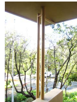
IMG_7015 steel pipe columns support porch roof
