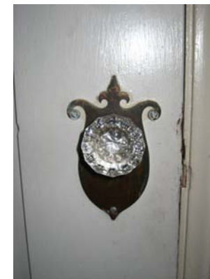
IMG_7245 crystal knob and bronze shield escutcheon
