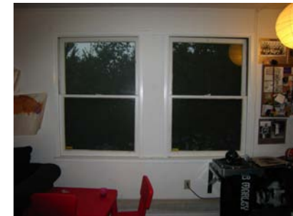
IMG_7103 paired double hung windows date from original dormitory room
