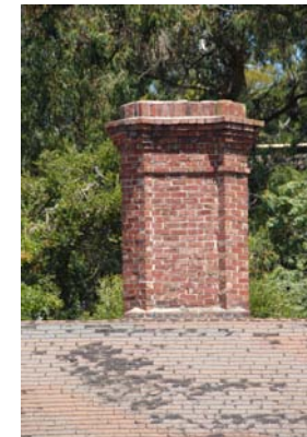
DSC_0080 corbeled brick chimney for kitchen
