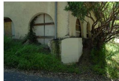
DSC_0089 damage and alteration at northwest corner; original arched openings at basement filled
