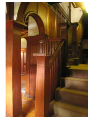
IMG_7250 bottom of stair showing redwood wainscot, curved rail, balustrade, and newel post
