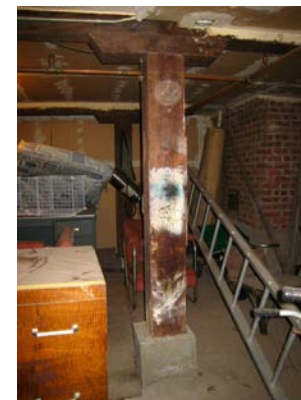
IMG_7901 wood beams and posts on concrete footings, looking north
