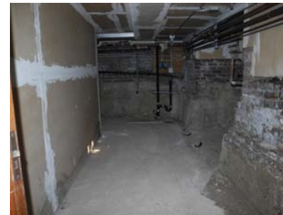
IMG_0791 gypsum board partitions and ceiling added as fireproofing measure
