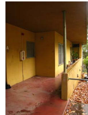
IMG_6896 Steel pipe post and rail, integrally colored concrete slab
