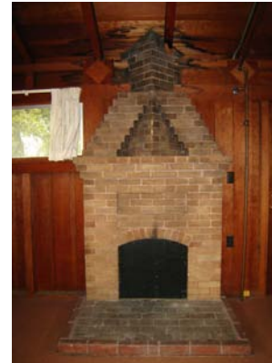
IMG_6714 corbeled brick chimney at north wall
