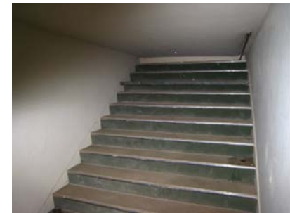
IMG_6875 interior stair to dormitory abandoned and upper floor infilled when dormitories were converted to apartments.
