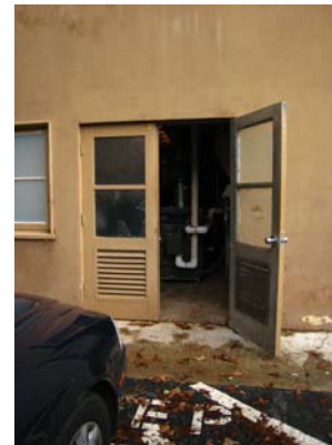
IMG_7057 original three panel doors on north elevation at basement mechanical room
