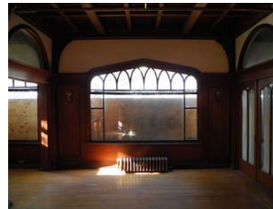
IMG_0716 west wall with Tudor arch window opening. Divided lights at top of window suggests intersecting tracery.
