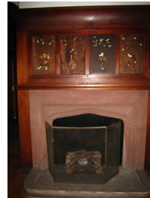
IMG_6710 carved red sandstone fireplace with Tudor arch opening and curbed hearth
