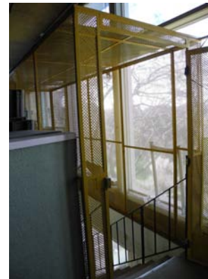
IMG_0857 Expanded metal grill cage and security door added at top of stair after original construction.
