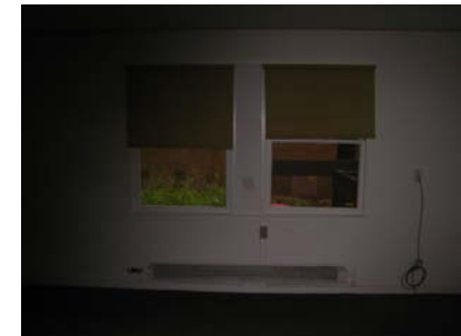
IMG_7190 baseboard radiator below paired double hung windows
