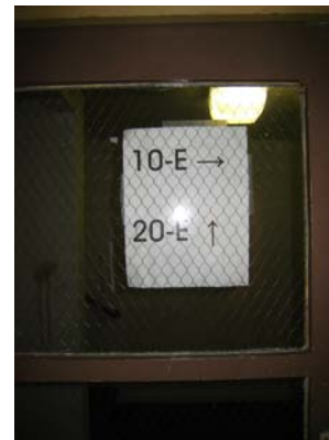
IMG_6865 detail of door with wireglass upper panels
