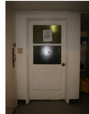
IMG_7055 original three panel door at storage room
