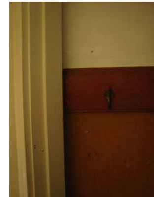
IMG_7848 hooks at redwood board picture rail with plaster finish above and paper finish below
