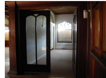
IMG_0718 paired glazed doors with divided lights suggesting simple tracery
