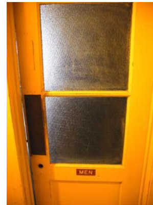
IMG_0866 historic three-panel door with textured glass upper panels
