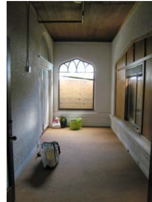
IMG_7263 small lights at top of window suggest intersecting tracery; new window added in original opening at right
