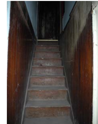
IMG_0799 redwood wainscot at back basement stair that leads to butler's pantry and exterior
