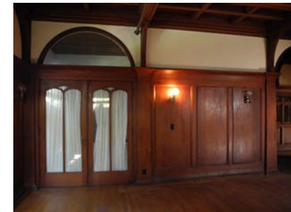
IMG_0717 north wall with glazed arch transom above paired glazed doors to porch. Divided lights in doors suggest tracery.
