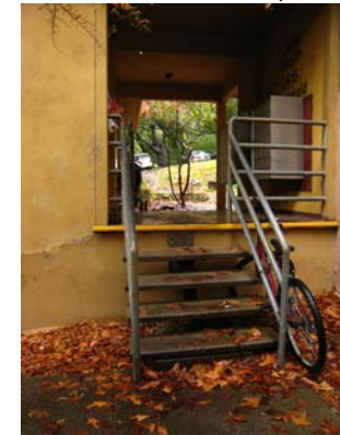
IMG_6905 steel pipe rail and steps
