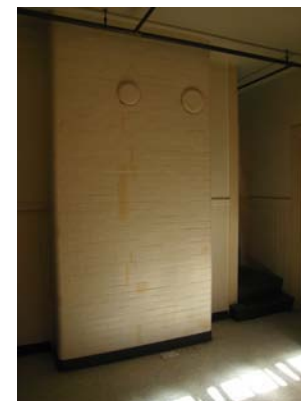
IMG_7276 brick flue at north wall
