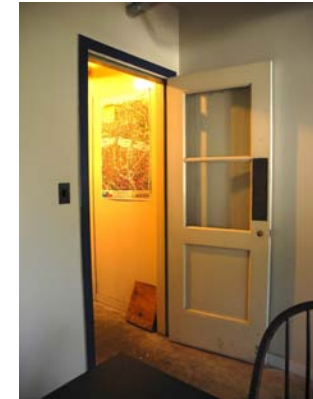
IMG_0864 historic three-panel door with glazed upper panels, looking southeast
