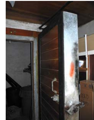
IMG_0817 wide insulated refrigerator door at east wall
