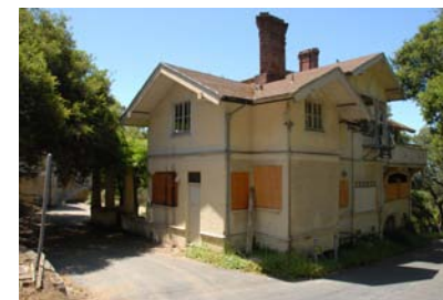
DSC_0085 northeast corner with cross gabled roofs, high decorative chimneys, and continuous water table at first floor.
