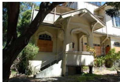
DSC_0096 entry porch with altered stairs and rail. Original arched openings at basement filled and altered
