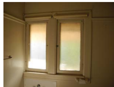
IMG_0766 textured glass in casement windows on west wall
