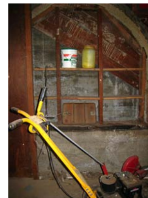
IMG_7898 Infilled arched openings at exterior walls
