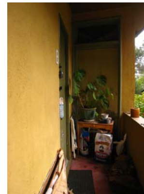
IMG_6916 original glazed openings infilled at entry area; solid door and double hung windows added
