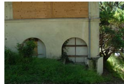
DSC_0088 arched openings at basement filled; alterations and damage at southwest corner
