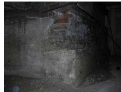
IMG_0792 brick and concrete foundation
