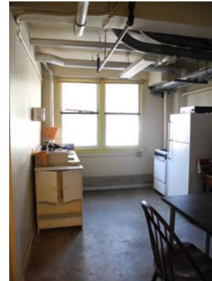
IMG_0863 paired double-hung windows on west wall
