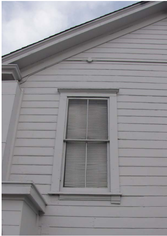
Figure 11: Detail of the original wood windows and wood siding.
